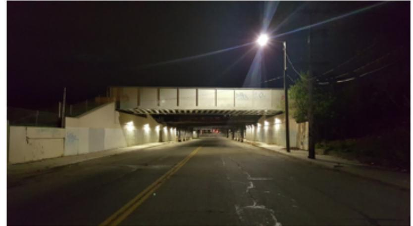
***This viaduct, one of several crossing Junction Street, is a good model for improvements to other viaducts: well-lit sidewalk and roadway area, stable and clean foundation walls, functioning drainage. Most other viaducts have multiple support piers between their abutments, requiring additional light fixtures to achieve consistent lighting levels.***
